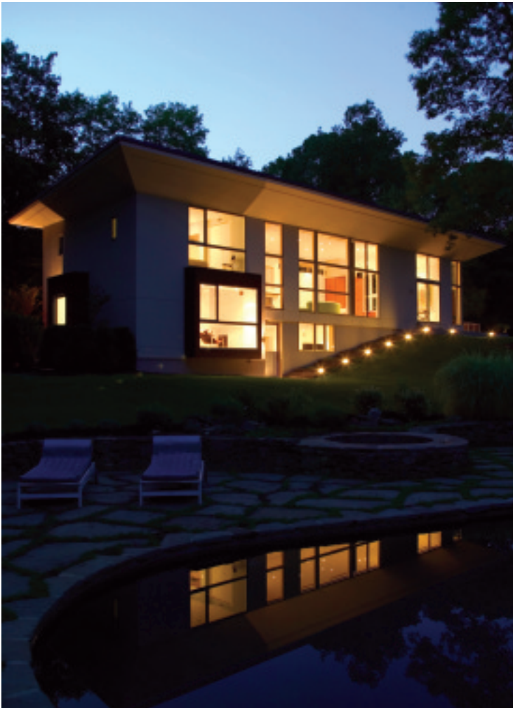
Photos Courtesy of Randy O'Rourke/Corporate Construction
